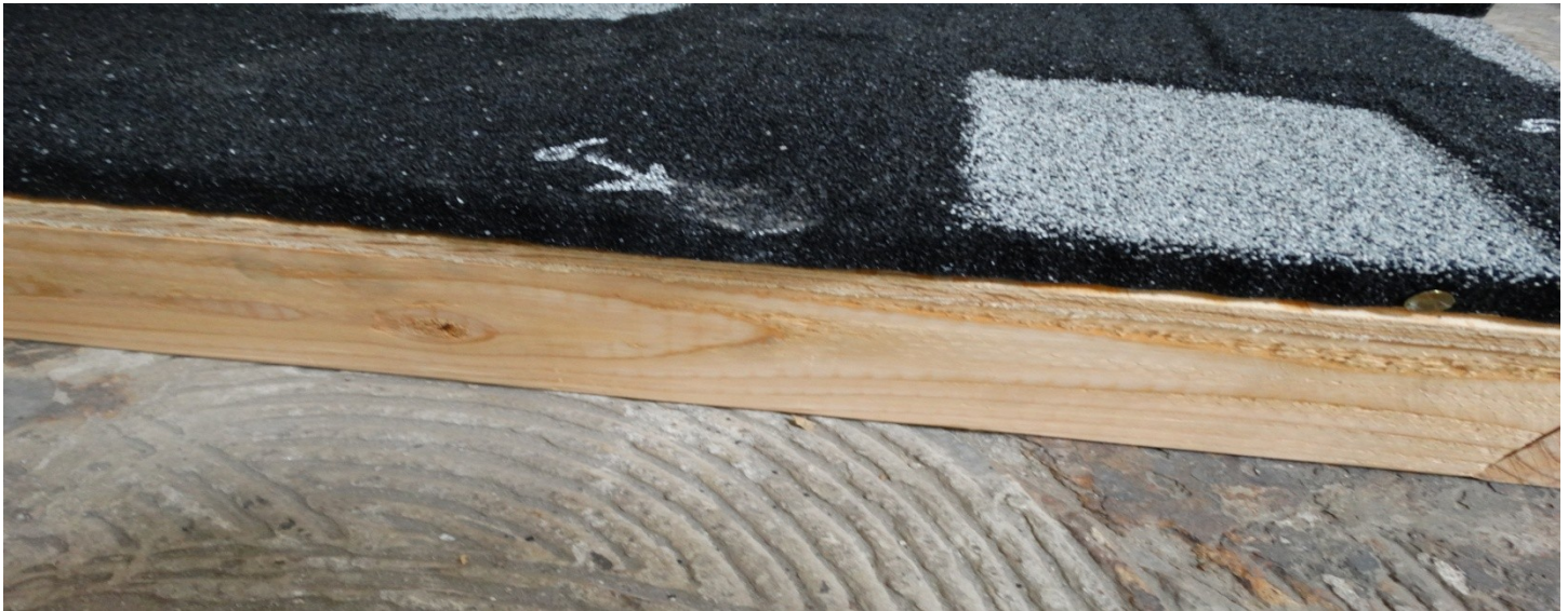
Photo 4: Drop 4 (Tile Joint), Drop 5 (Tile Corner), Drop 6 (Tile Edge).
